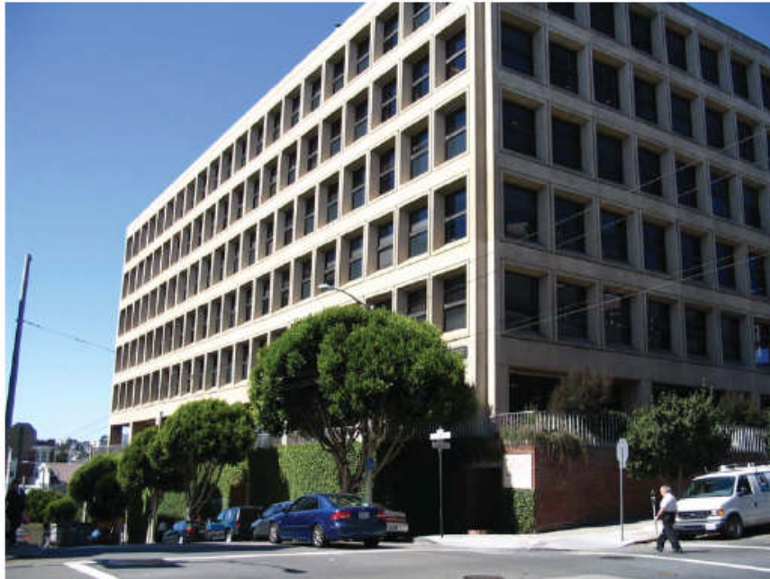
Photo 1 School of Dentistry Main Facility
