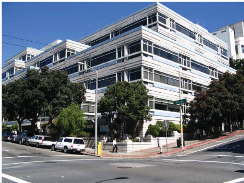
Photo 2 CPMC Medical Office Building - Northwest corner of Sacramento and Webster Streets
