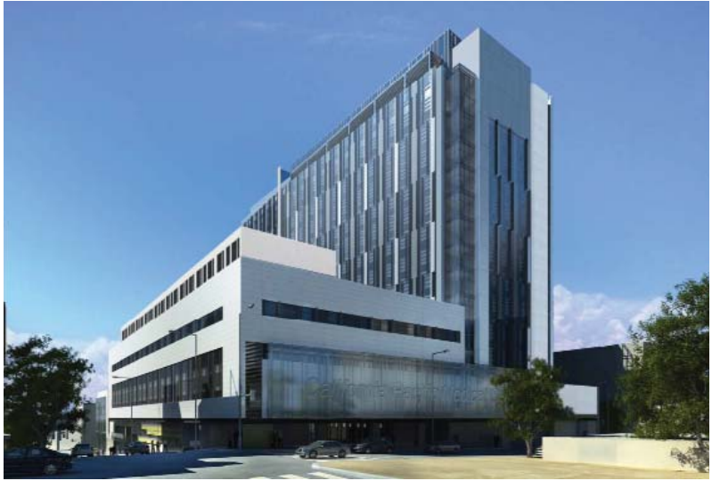
View of emergency department entrance from Franklin and Post.
