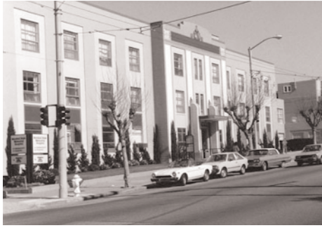
Marshall Hale Hospital, c. 1974
