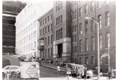
L to R: 2333 Buchanan under construction, Stanford Building, Lane Building, c. 1971
