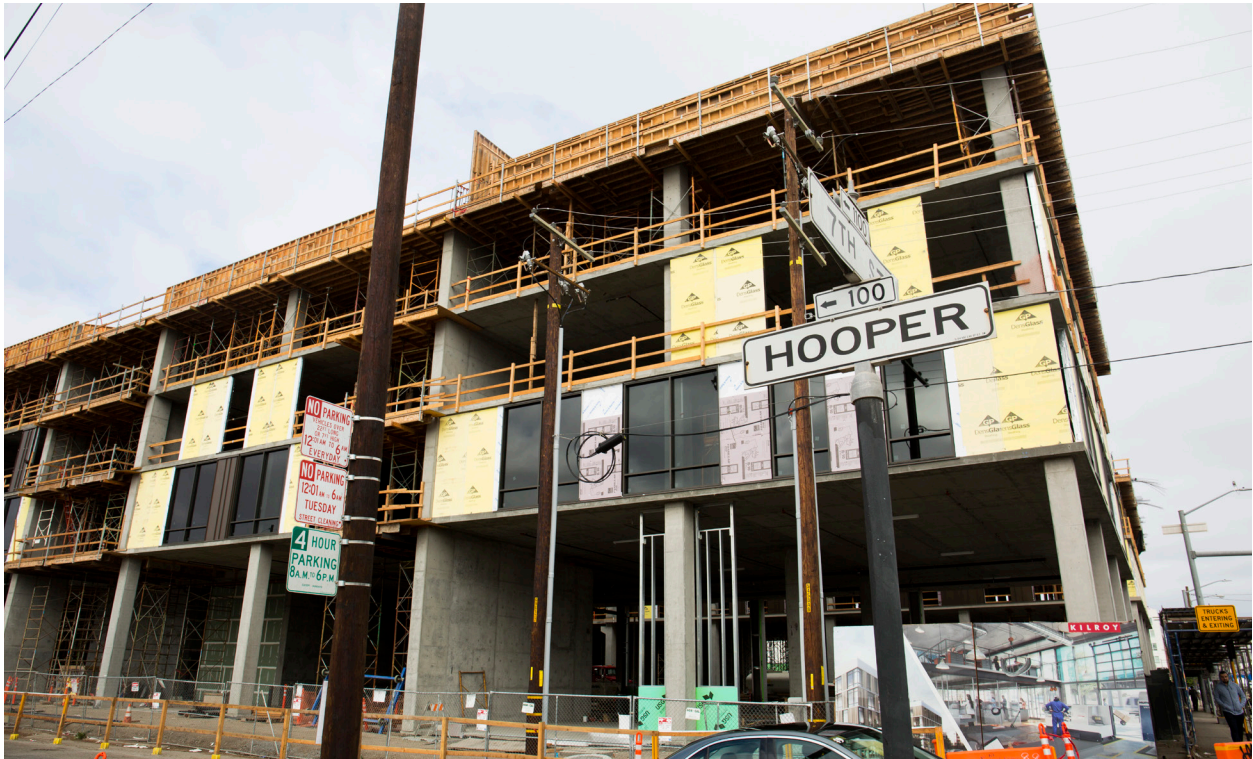
Neighboring business at 7th and Hooper looking North
