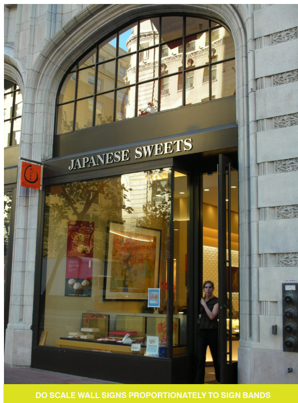
This wall sign is centered on the storefront, scaled proportionally to sign band and does not alter any character-defining features. This treatment is recommended.
