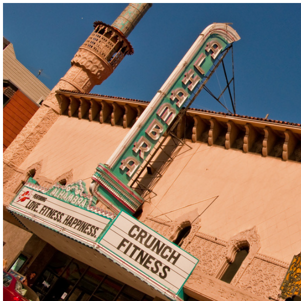
Example of a historic movie theater sign
