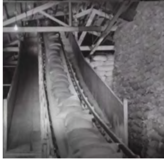
Chute down off dock
