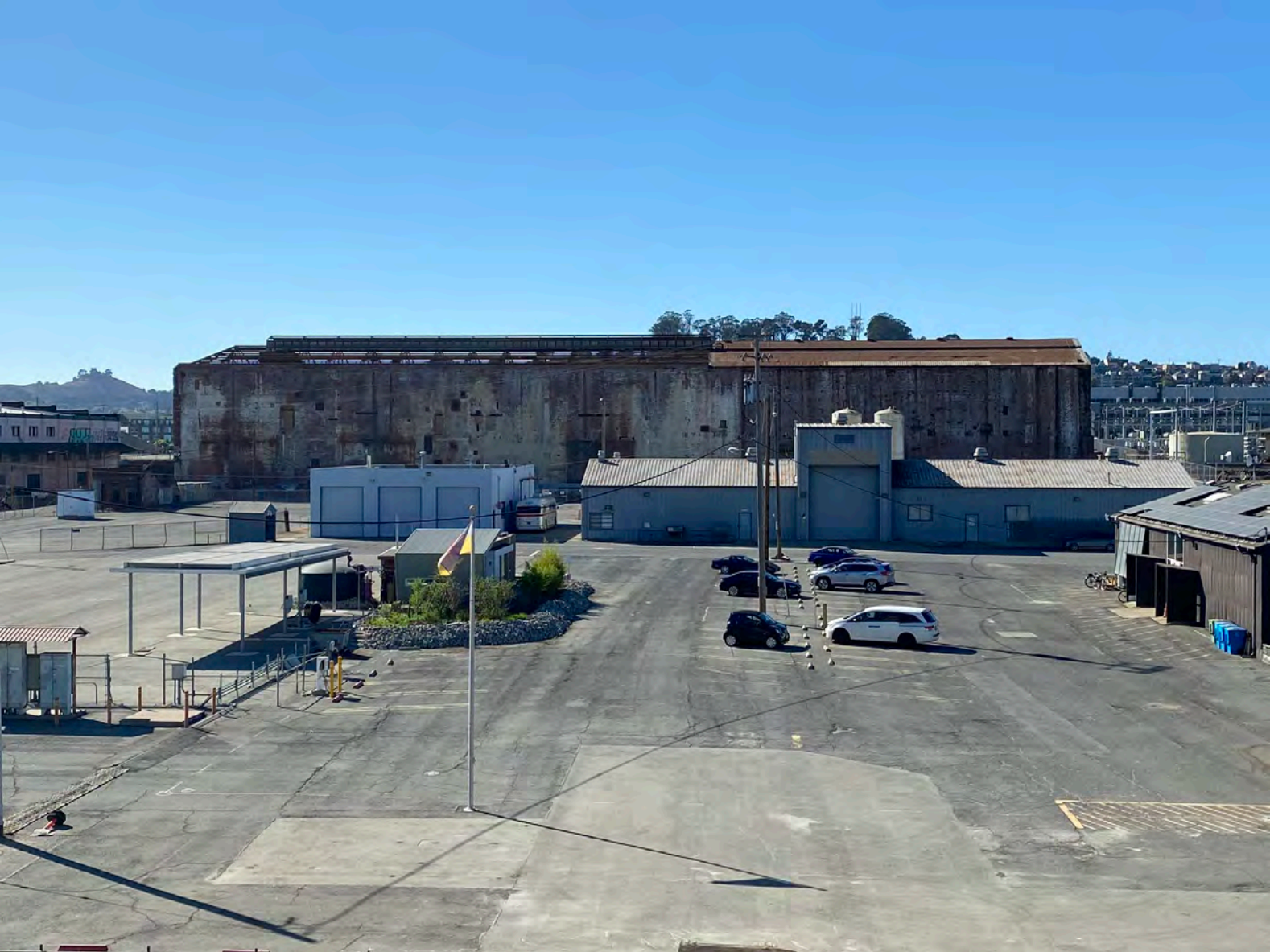
View of existing conditions looking west.
