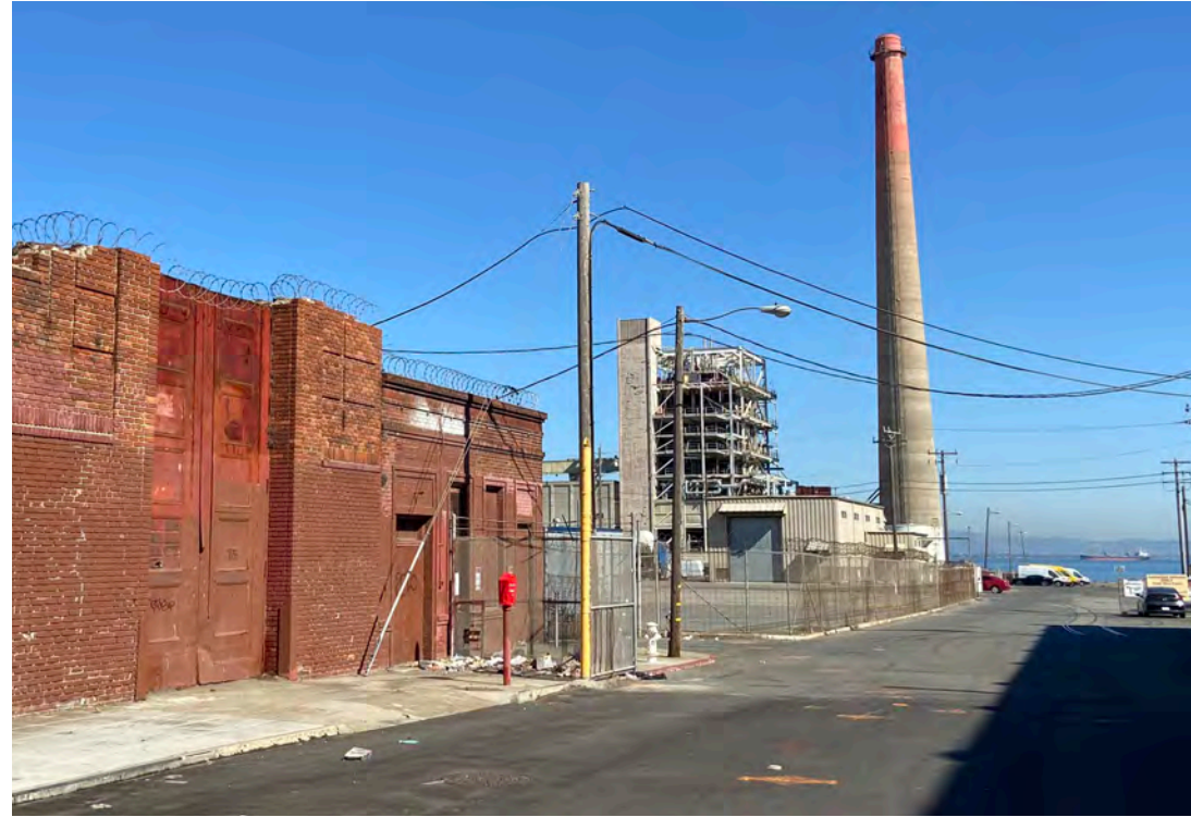
Boiler Hall Metal Panel Doors
