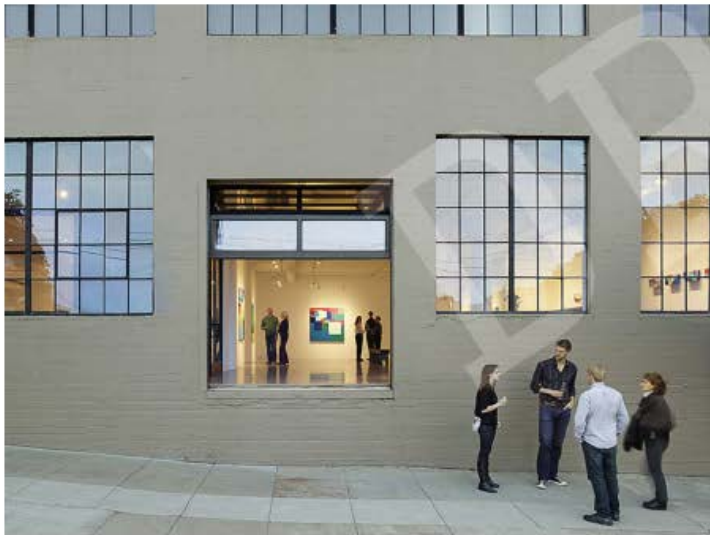
Organize internal uses and reconsider building openings in creative ways to connect to exterior spaces.
