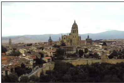
Walls of Segovia, Spain
