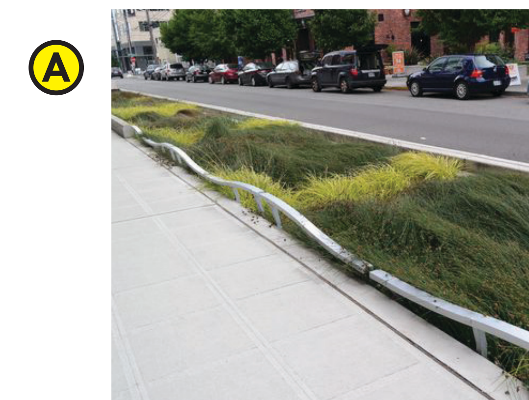
A RAIN GARDEN A linear raingarden would extend the green space from the park down Octavia Boulevard and into the neighborhood
